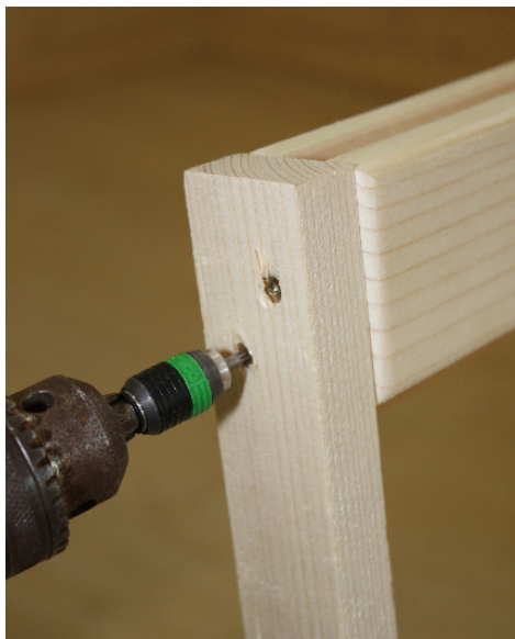
Remove transport strip from the door frame
