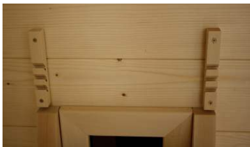
Fig. 47: Installation of the headrests
