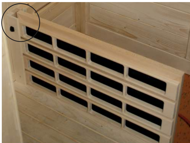
Fig. 32: Installation of the IR thermal plate VitaMy 164
