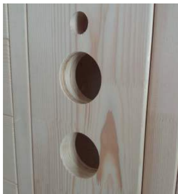
Fig. 43: Installing the control panel
