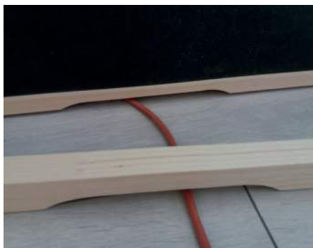
Fig. 33: Inserting the stiffener bar for the Vitamy IR thermal plates.
