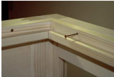
Fig. 14: Roof support slats installation
