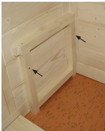
Fig. 30: Installation of the bench cushion
