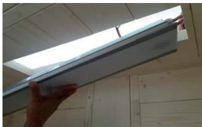
Fig. 44: Installing the colour light
