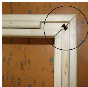
Fig. 2: Connect the floor frame elements
