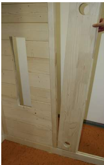
Fig. 6: Install the electrical element in place
