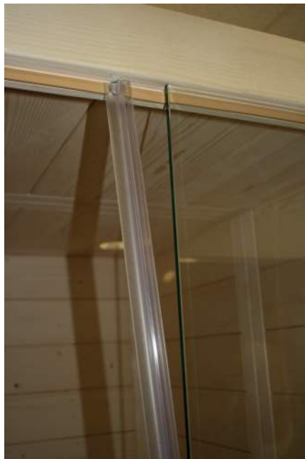
Fig. 19: Installing the door insulation strips
