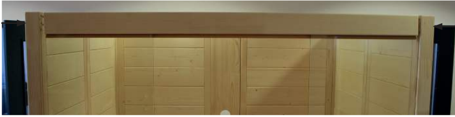
Fig. 13: Attaching the skirting
