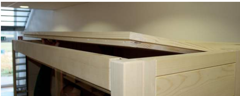
Fig. 17: Installing the roof element in the front
