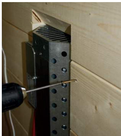
Fig. 37: Installing the rear radiator blind
