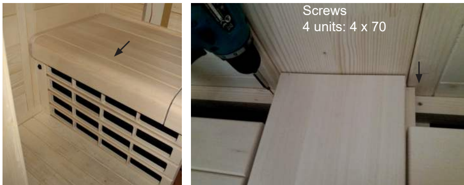
Fig. 45: Attaching the bench
