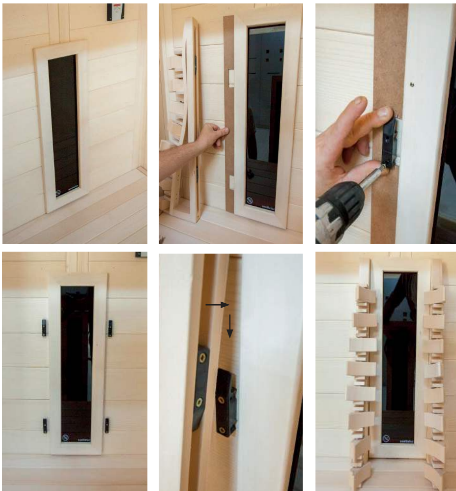
Fig. 29: Installing the backrests
