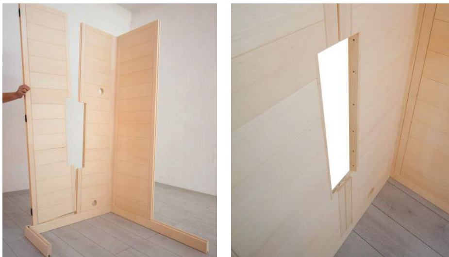
Fig. 6: Inserting wall element with recess
