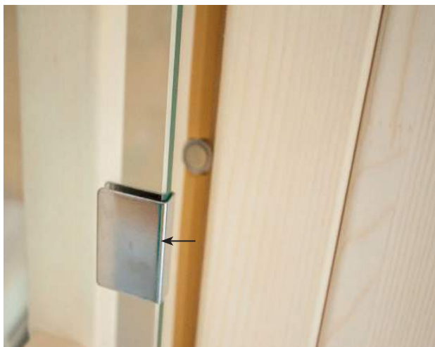
Fig. 35: Assembly of sleeve plate
