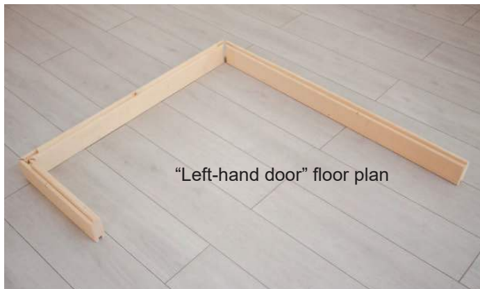
Fig. 1: Laying the three base frame elements
