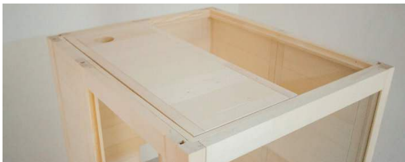
Fig. 14: Inserting front ceiling element
