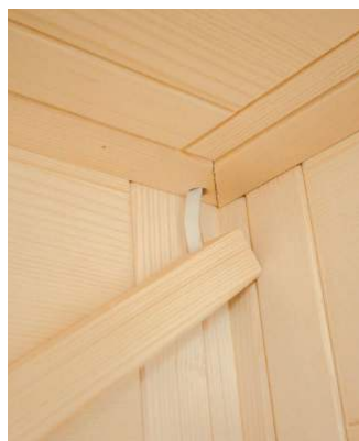
Fig. 24: Fixar a barra LED
