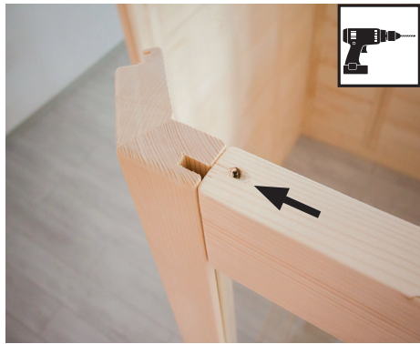
3 mm drill bit, 1 screw 4 x 70 mm
