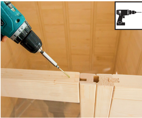
3 mm drill bit, 1 screw 4 x 70 mm
