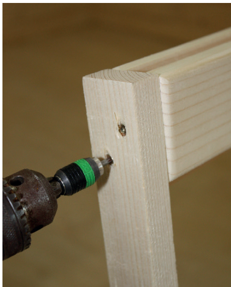
Remove transport strip from the door frame
